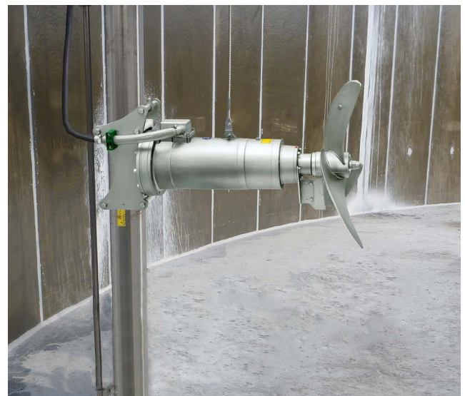
3A - Steel tank
