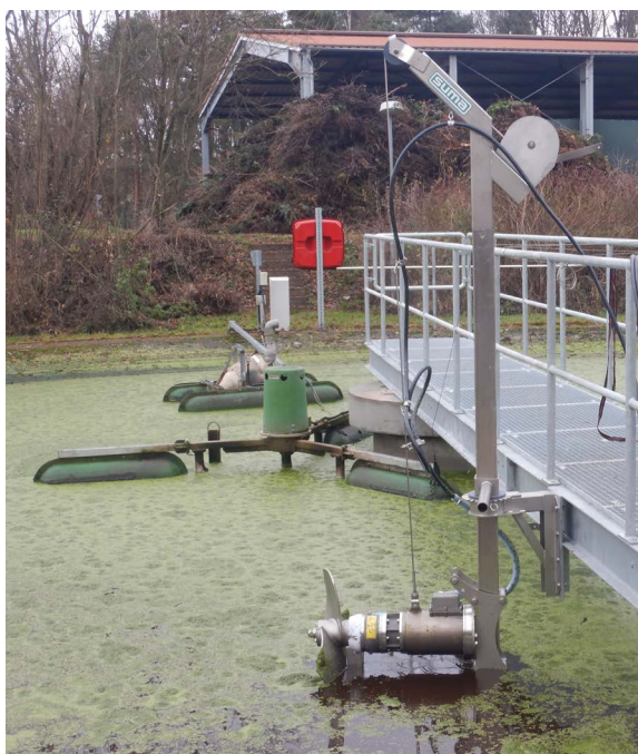
2A with EV - Open tank
