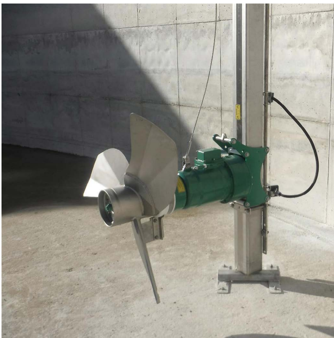
4G with EV - Closed tank
